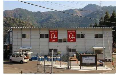
Hibigatani Waste and Resource Station
