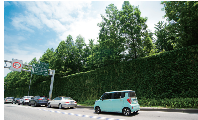
Soundproof wall to prevent traffic noises
