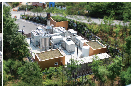
MCFC-type fuel cell station in Sangam (2.4 MW)
