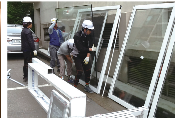
Window Reinstallation for BRP
