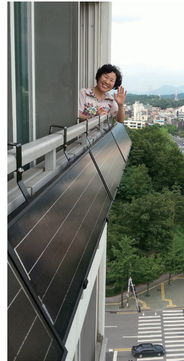
Mini PV System for Apartment
